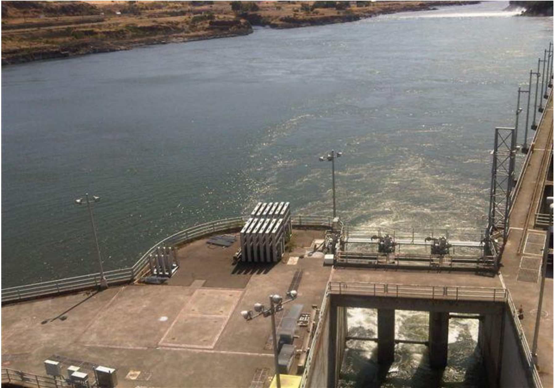
Attraction flow at the east entrance with Main Units 17 to 22 out of service for powerhouse roof contract. Previously coordinated through FPOM.
